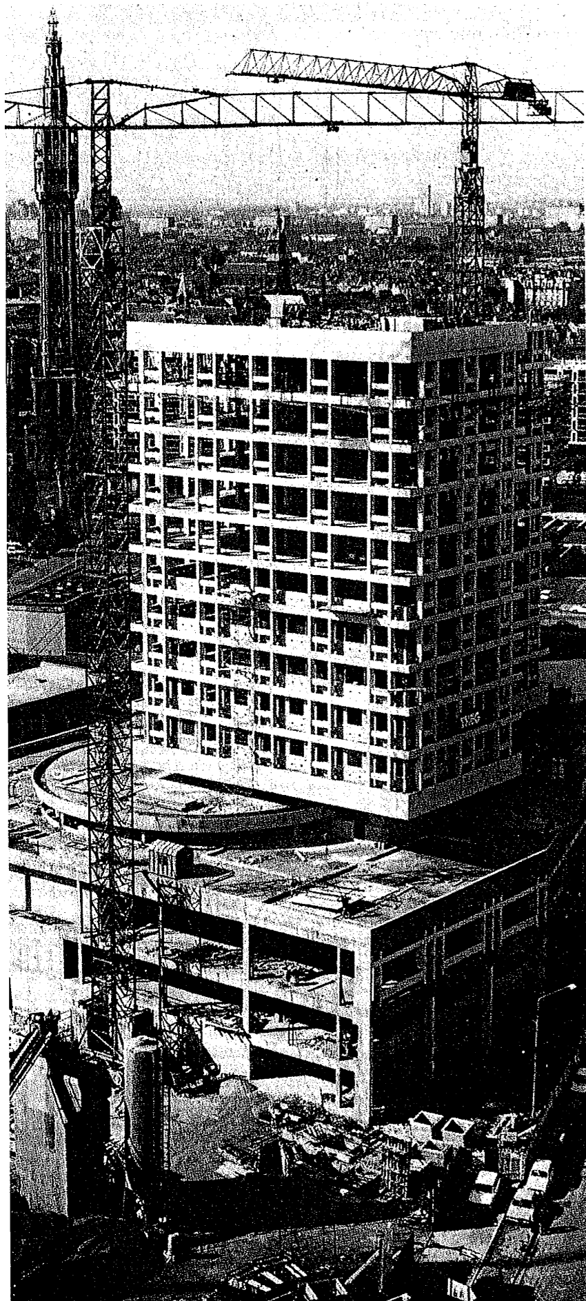
Ossature – Poteaux – Poutres – Planchers – B.A.
